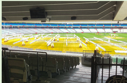
There are shaded areas during the day therefore, to make the grass grow, heated lights are used.
